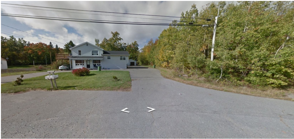
Figure 7 – Commercial / Residential Building (Wolfville Ridge)
