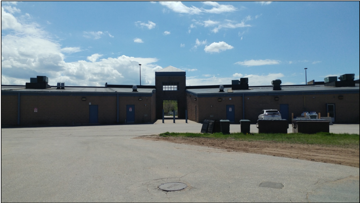
Figure 3 - Greenwood Mall, Facing Subject Property
