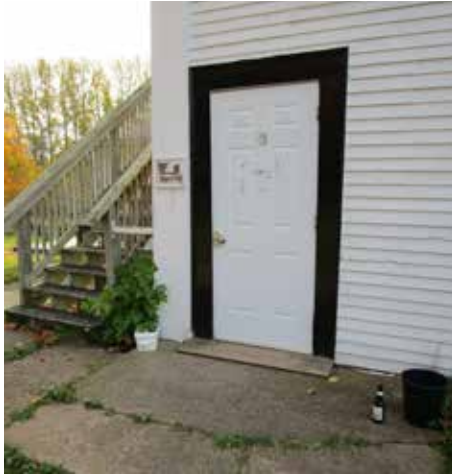
KA 10 | Accessible entrance to Sheffield Mills Community Hall
