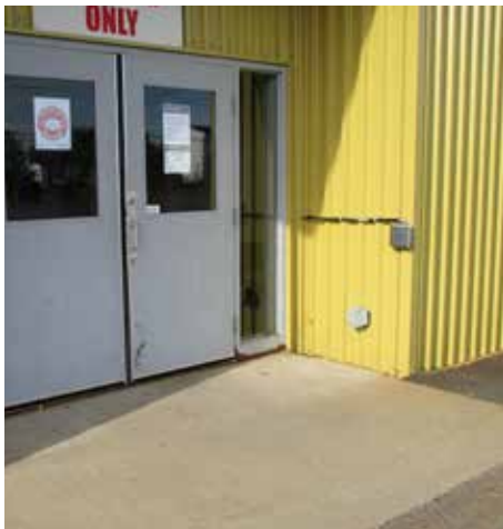
KA 6 | Power Door Control at Entrance
