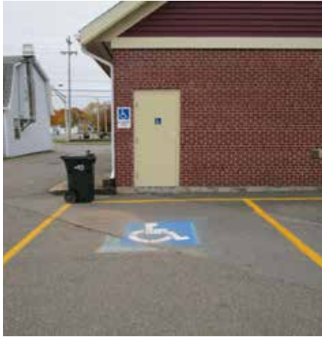
PA 7 | Accessible parking at the back of the Kentville Village office
