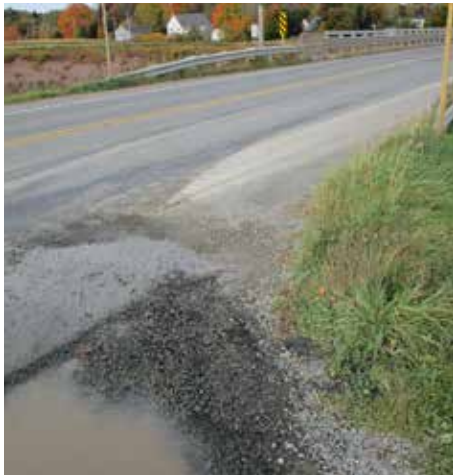
PS 2 | Pot holes leading to Port Williams bridge
