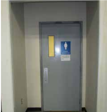
WS 4 | Womans washroom door at Glooscap Arena.
