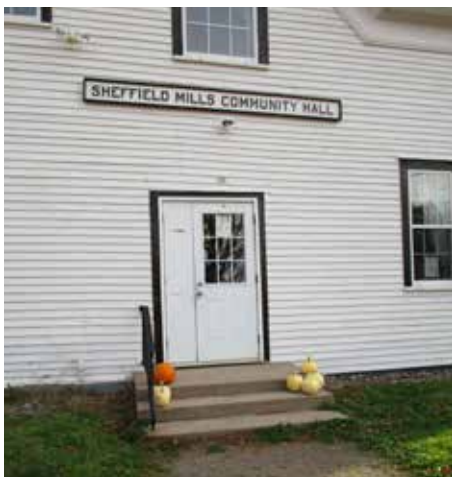
KA 9 | Stairs leading into the front entrance of the Sheffield Mills Community Hall
