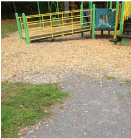
KA 14 | Entrance path to accessible playground in Centreville
