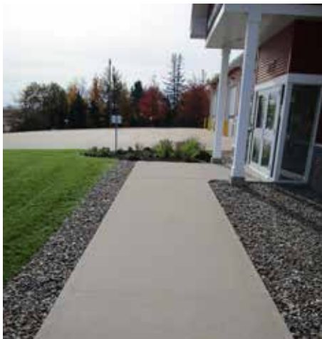
KA 8 | Pathway leading to the Canning Fire Hall
