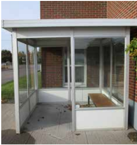
TR 2 | Bus Stop in Port Williams, No accessible space not in path of travel
