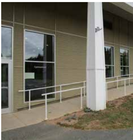
KA 12 | Exterior ramp to access interior rooms within the village office
