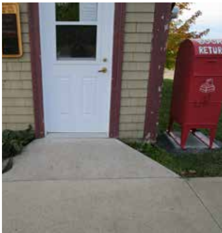
KA 3 | Canning Library with sloped access and inaccessible book return
