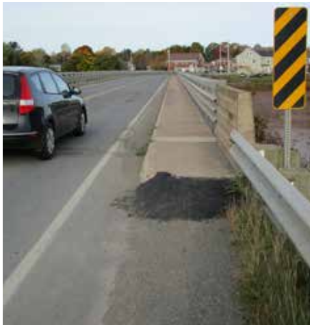
PS 3 | Ramp to path on Port Williams bridge
