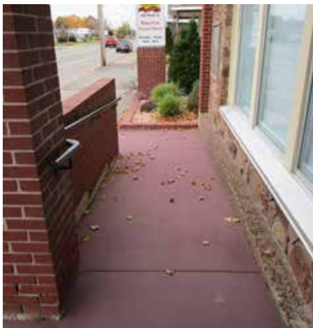
KA 19 | Ramp leading away from entrance
