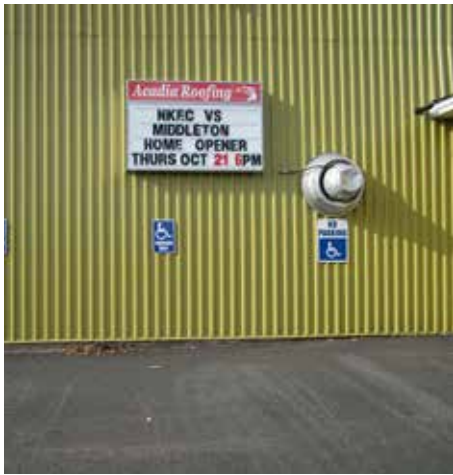
PA 5 | Accessible parking signage at Glooscap Arena
