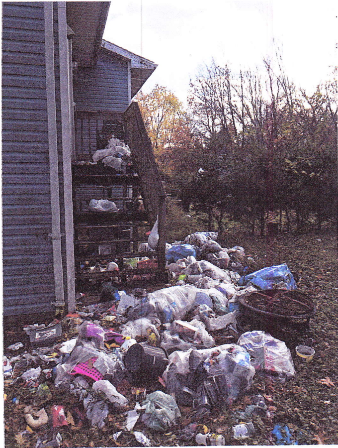
Waste accumulation at a rental house (owned by Housing Authority).
