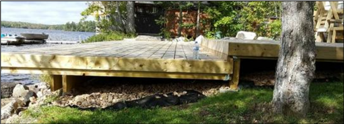
Figure 2: Two-tiered deck following the natural slope and integrating porous materials
