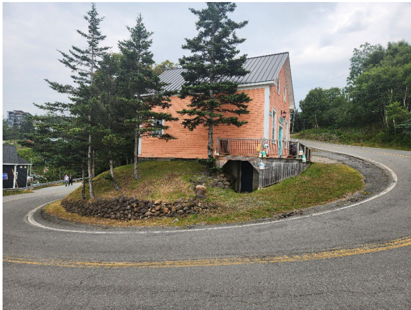
Figure 3: Subject property and building
