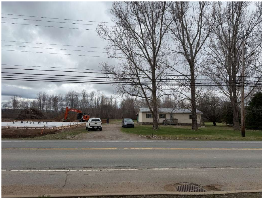
Image 4: Looking at the site and existing driveway. The development seen on the left is an adjacent property under different ownership.
