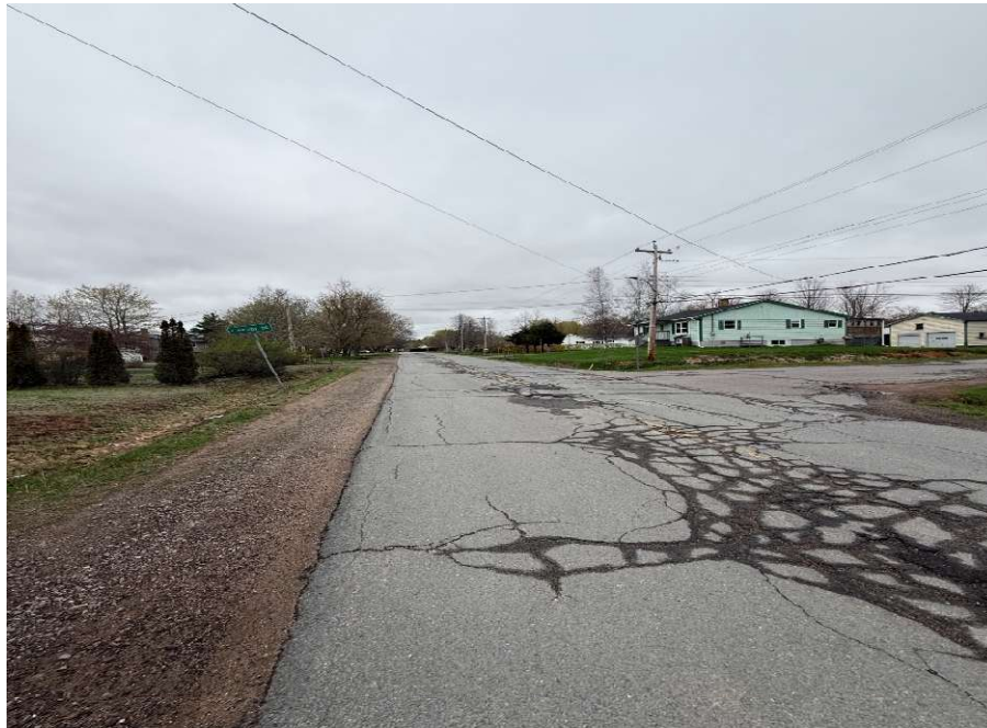
Image 2: Looking west from the subject property towards Sherman Belcher Road.
