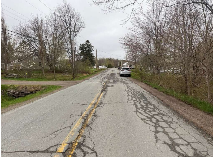
Image 3: Looking east from the subject property towards Highway 359.
