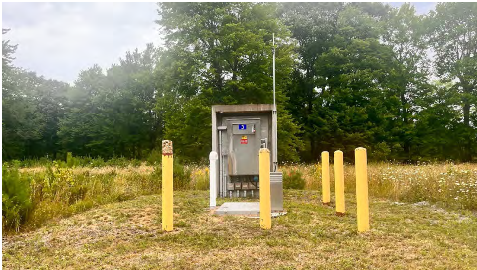
Photo: Sewer lift station on the corner of Central Ave and Bedford Road.
