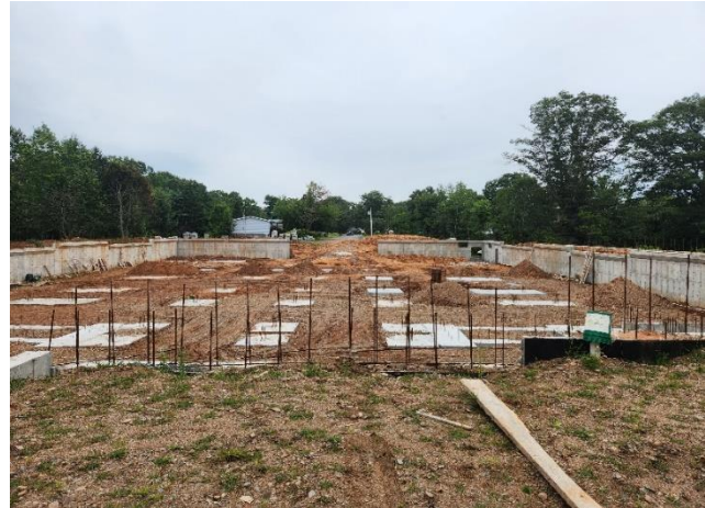
Figure 2: View of the Subject Property
